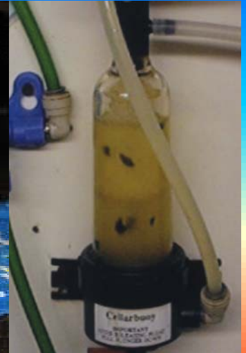
J Pull off 1 litre of cleaning fluid and examine for alien objects. (However, allow for the fact that the fluid is naturally cloudy.)
